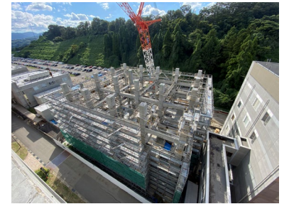
躯体工事 (R6.9)
